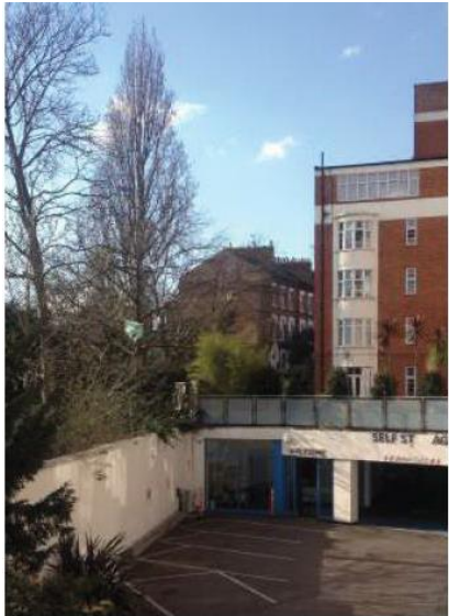
2 House 1 Existing View from William Court Service Entrance
