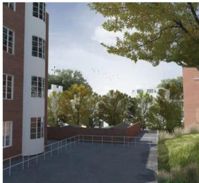
2 House 1 Existing William Court Podium View
