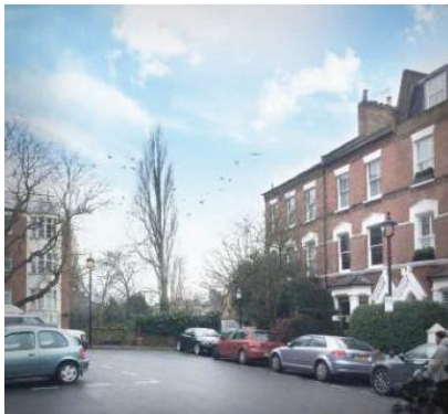
House 1 Existing View from Hamilton Gardens
